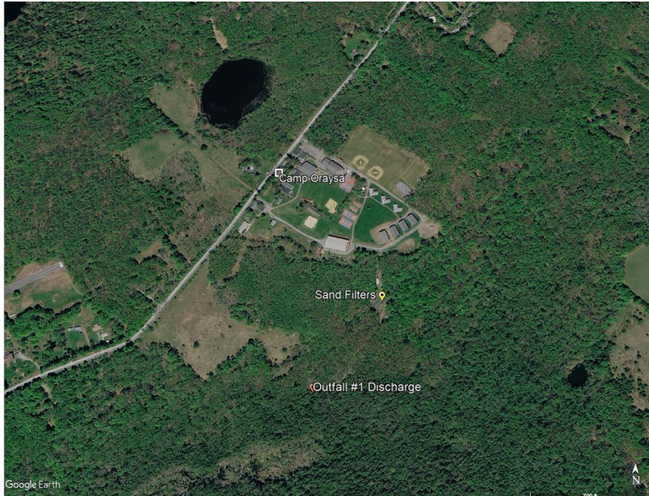
Figure 2. Camp Oraysa Outfall and Sand Filter Locations.
